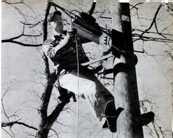
Signal that a new phone is on the way—Charlie Thomas, installer for the N. Y. Telephone Co., connects wire that goes to the house to one (called a "pair") that goes to the exchange.
